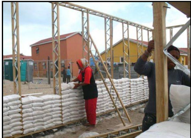
FIGURE 8c: Construction of a wall using wooden beams and sandbags, Sandbag Houses , Freedom Park, Cape Town, 2007.
