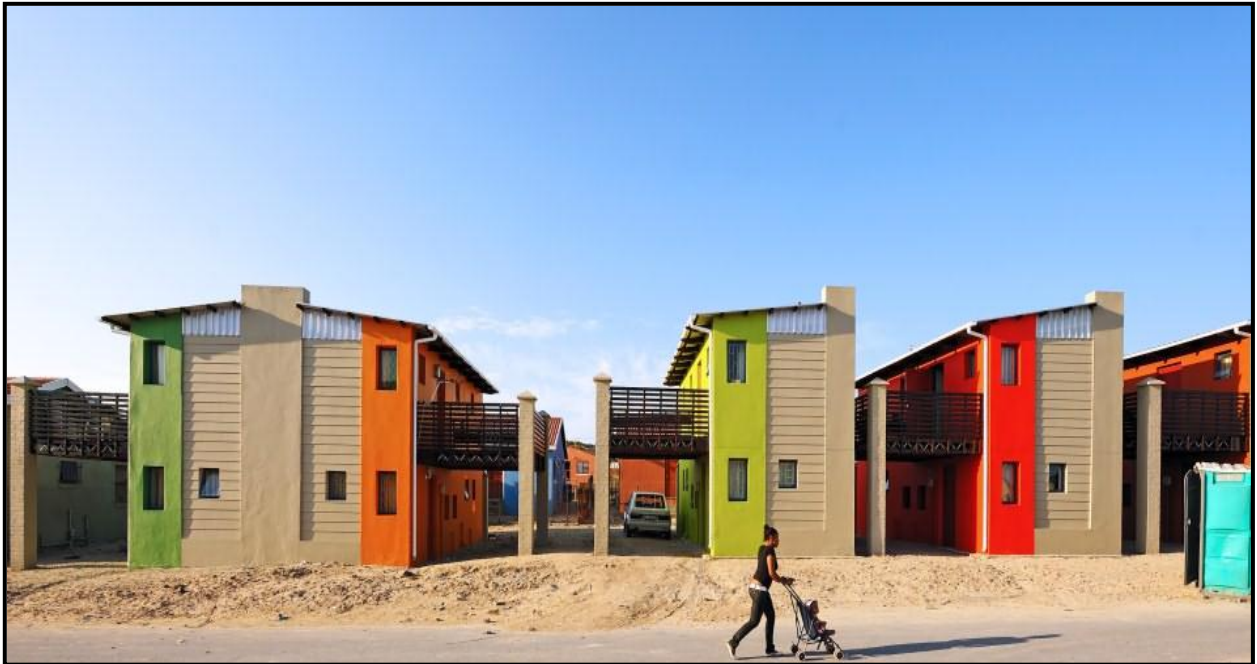
FIGURE 8a: MMA Architects, Sandbag Houses , Freedom Park, Cape Town, South Africa, wooden beams and sandbags, 2007.
