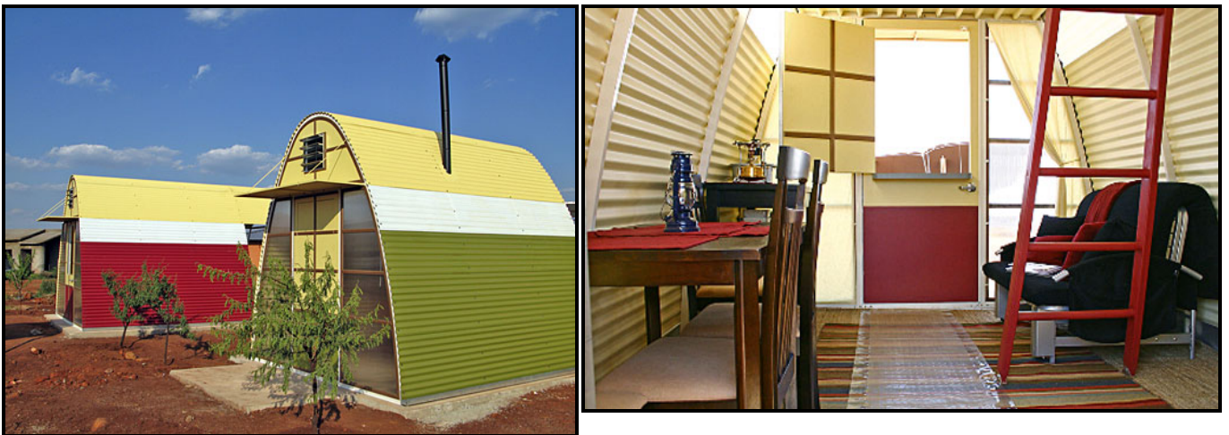
FIGURE 8b: BSB Design, Architecture for A Change, (AFAC) . Prototype for the use of affordable/micro-housing in South Africa, solar panels, corrugated metal, glass, 2013. (Exterior and interior views)
